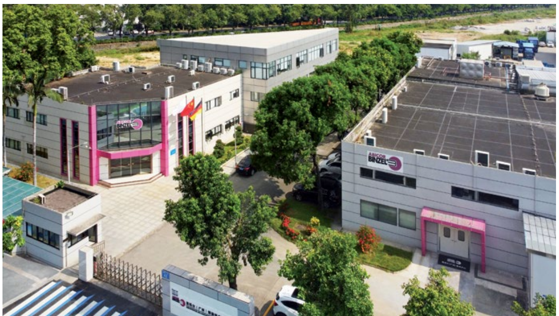
Building complex ABICOR BINZEL (Guangzhou) Welding Equipment Co. Ltd.
