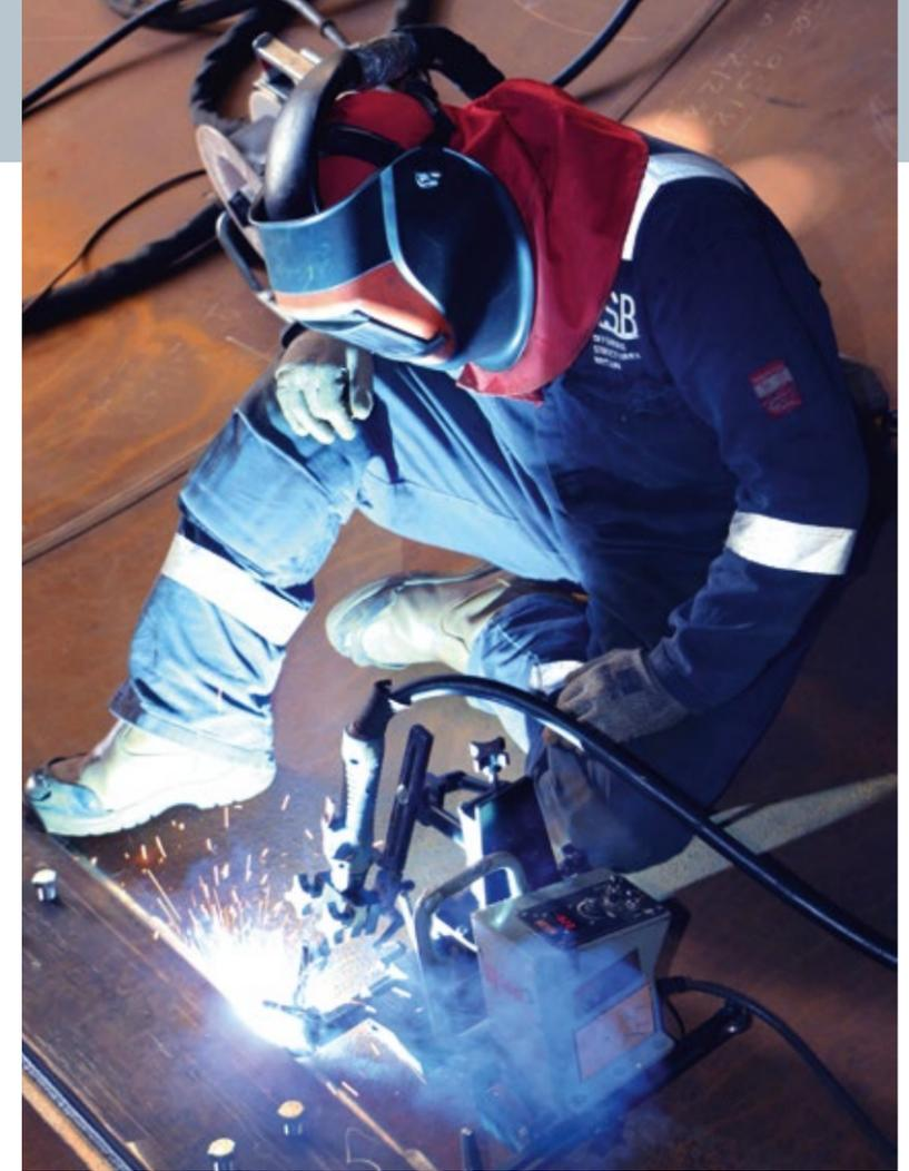
reduced weight cable assembly of the air cooled ABIMIG® A T LW (low weight) torches are really beneficial for the welder.
