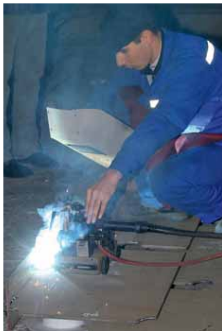
Support for welding long seams.
